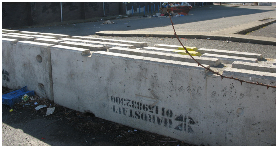
Interlocking concrete blocks but each may need to weigh up to 4.5 tonne
